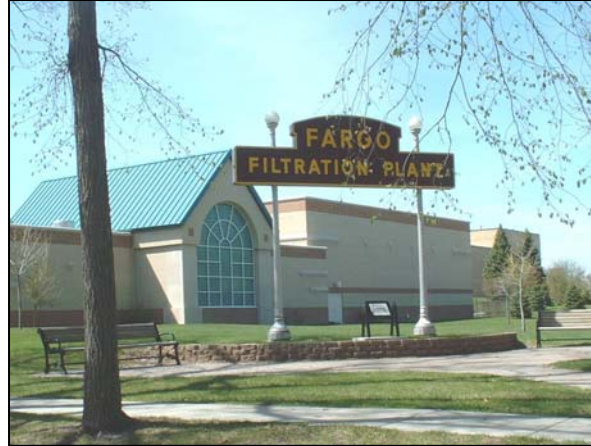
Fargo Water Treatment Plant
