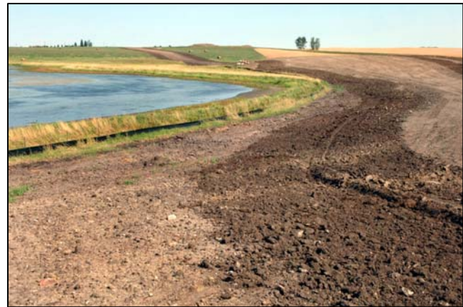
Wetlands Would Be Avoided by Pipeline Construction Where Practical and by Above-Ground Facility Construction.
