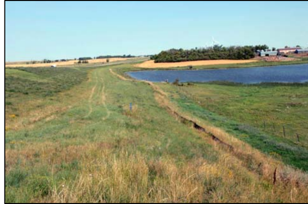
Post-Construction Overview of MR&I Pipeline
