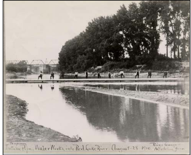
Grand Forks Water Supply Intake Pipe Exposed in the Red Lake River, a Tributary of the Red River, During Low Flow on August 28, 1910 (Photo Courtesy of Grand Forks)
