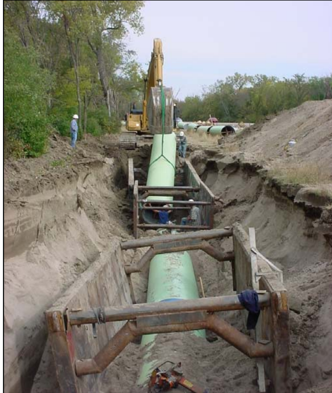
Construction of a Water Supply Project in South Dakota
