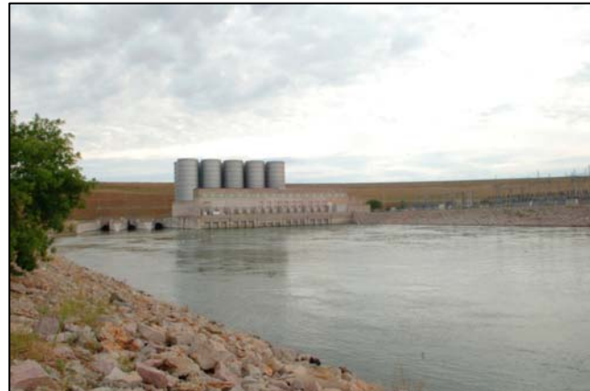
Garrison Dam Tailrace
