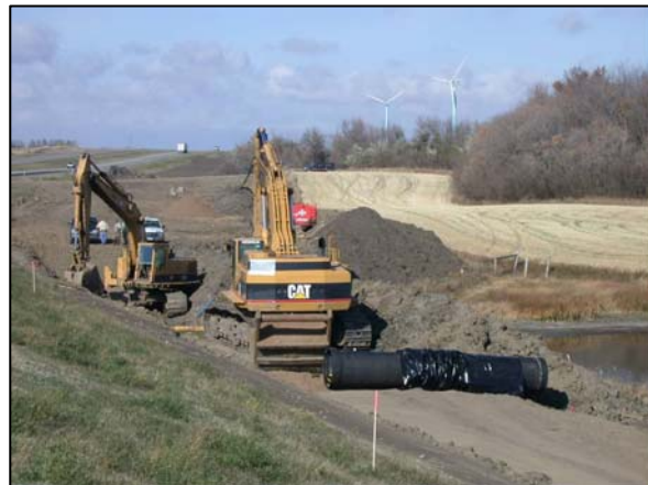
Pipelines Will Be Constructed Adjacent to Highways and Roads Where Practical.
